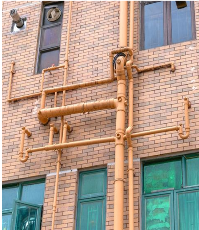
External wall of the building
